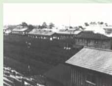
New school building in Koganei
